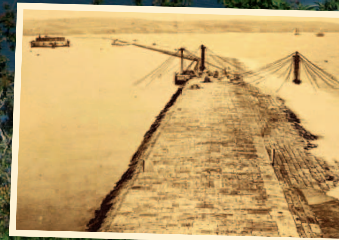
BELOW: The breakwater under construction.
